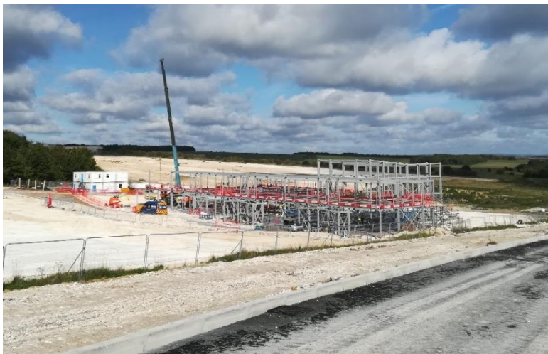
St. Michael's School build progress, Larkhill.
